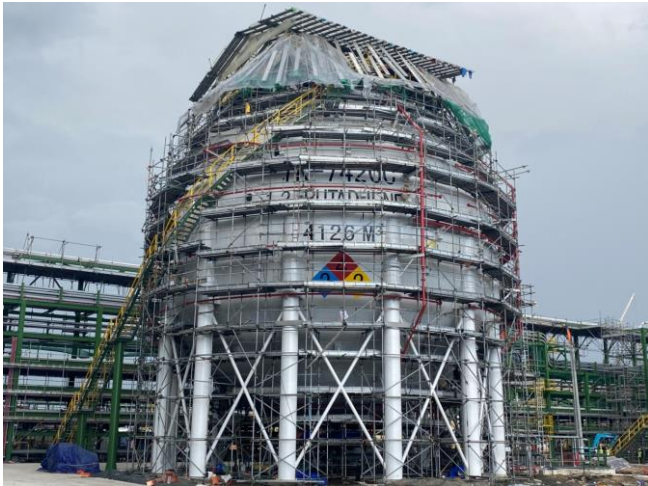
Insulation on spherical storage tanks in Vietnam
