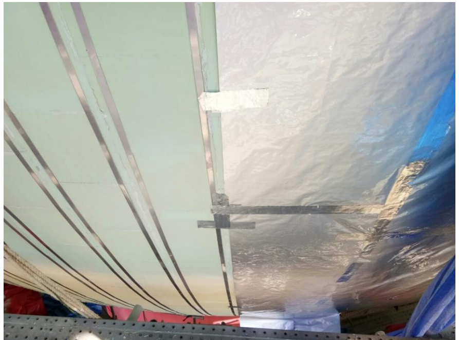
Stages of insulation on spherical tanks
