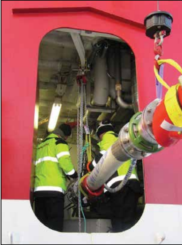
Connecting 6" Cryogenic Coupler and Breakaway
