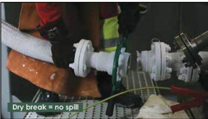
Disconnecting 3" Cryogenic Hose
